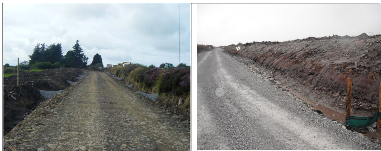
FIGURE 1 EXAMPLES OF CHECK DAMS AND EXAMPLE OF SILT FENCE USED IN CONJUNCTION WITH CHECK DAMS ALONG ROADSIDE DRAINAGE CHANNELS
